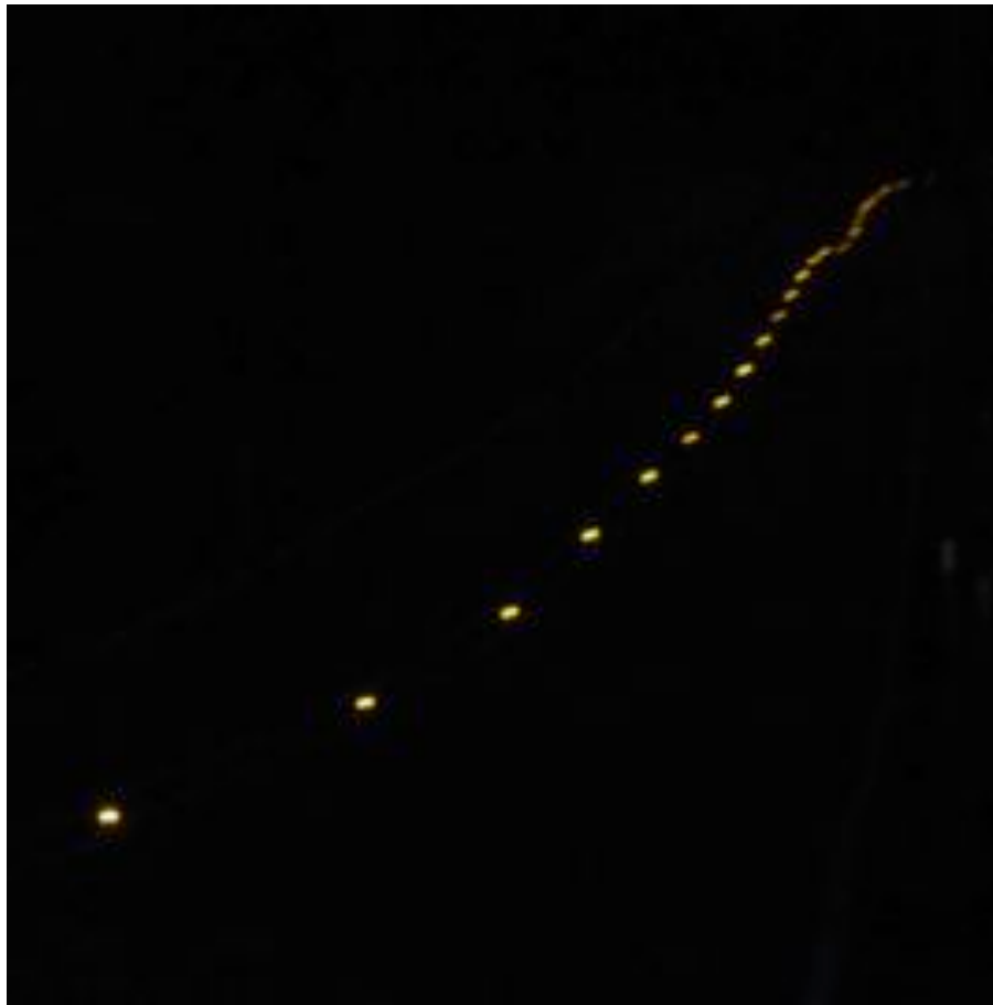
Figure 1: WSDOT - SR 530 – 900 plus feet of no passing zone with undulating terrain; Astucia flush studs milled-in subsurface on 40' centers
