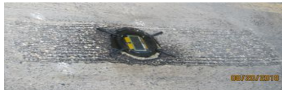
Figure 7: Milled-in Astucia flush stud
